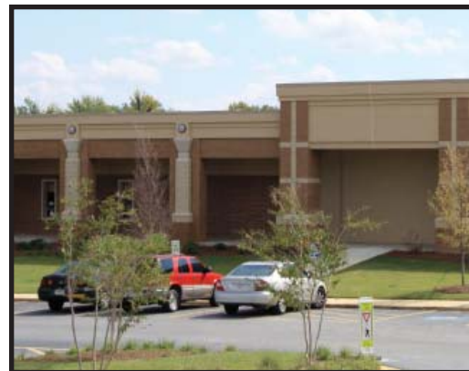
New facade for Building B at Macon Campus
